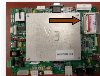
Figure 3 - Picture of the inside Vilter Panel
