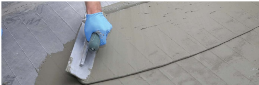
FIGURE 2.21: Install tile/stone flooring
