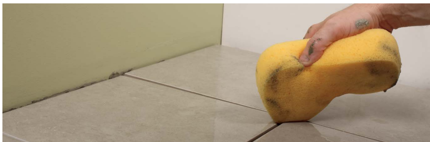
FIGURE 2.23: Clean grout lines
