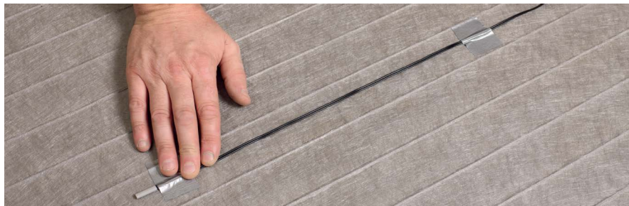
FIGURE 2.16: Secure floor sensor probe
