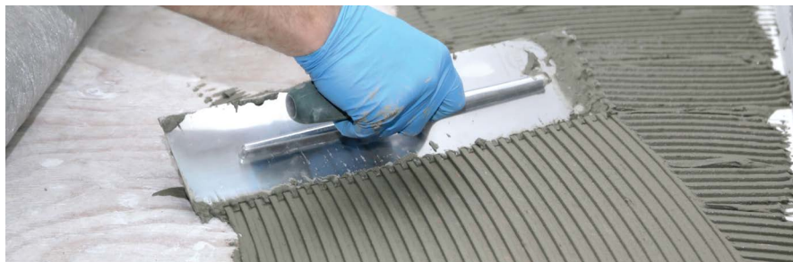
FIGURE 2.12: Spread thinset onto subfloor
