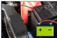
1.Power on to check light
