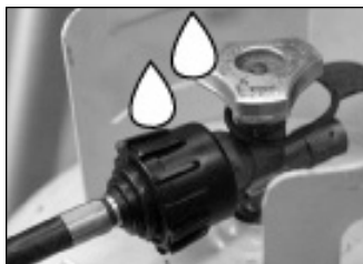
Leak Check Regulator & Hose
