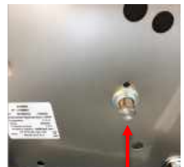
Remove Drain Plug (figure 2)
