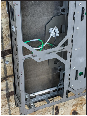
Figure 8: Install Power Entrance
