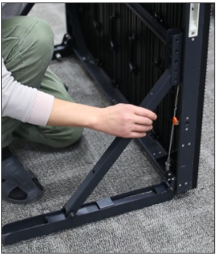
Figure 13: Extend Stiffeners
