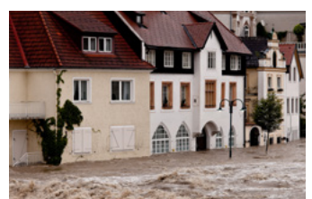
Water Damage Restoration
