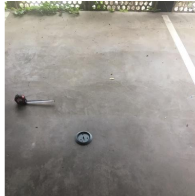
Figure 13 Sensor base installed
