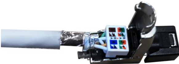
7.Place wiring cap on plug
