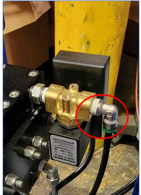
Figure 2. Typical diesel engine or electric motor compressor installation.
