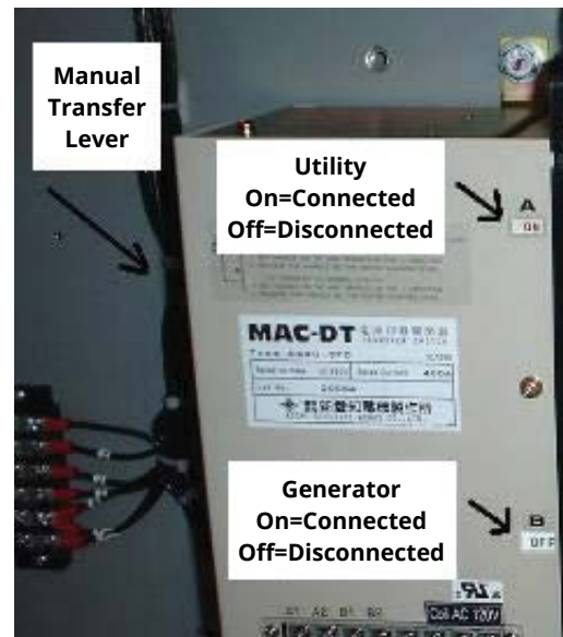
Figure 11 - Manual Transfer Lever Locations
