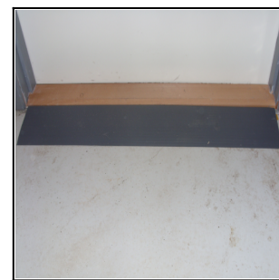
Ramp ready for use
