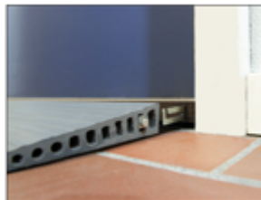
Mounting bracket mounted into the doorstep
