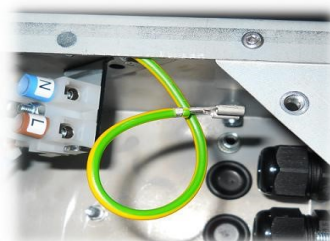
Fig.7 Grille Earth lead
