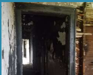
Fire Damage Restoration
