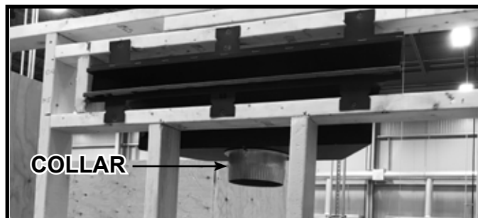
Figure 5.25 Install Collar(s) to Bottom of Plenum
