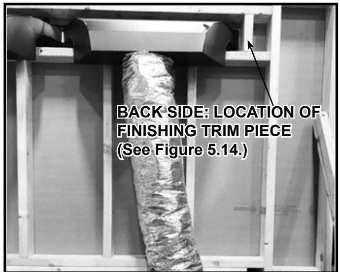
Figure 5.29 Flex Vent Installed with No Kinks
