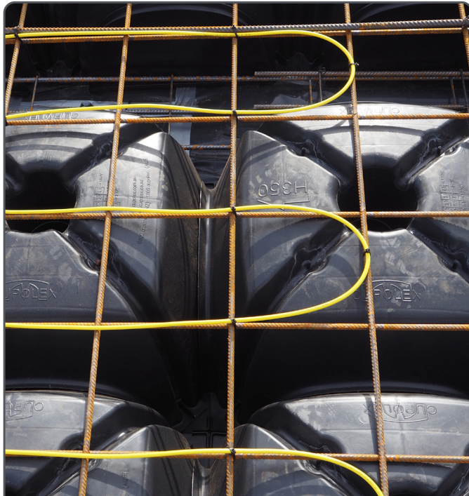
Secure the cables at regular intervals to ensure cables are held in place
