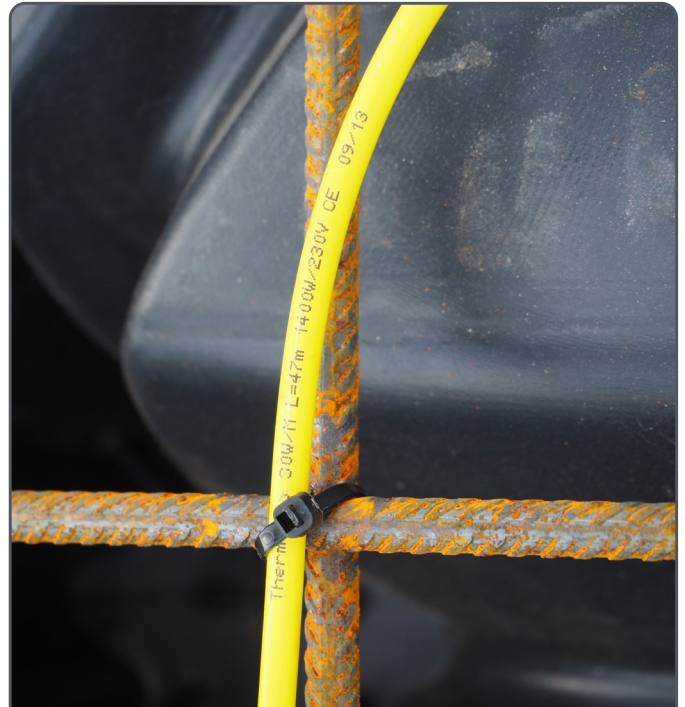
Cut the ends off the cable ties to ensure these do not protrude from out of the slab
