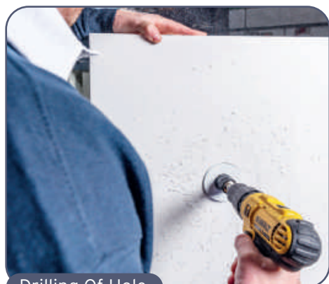
Drilling Of Hole
