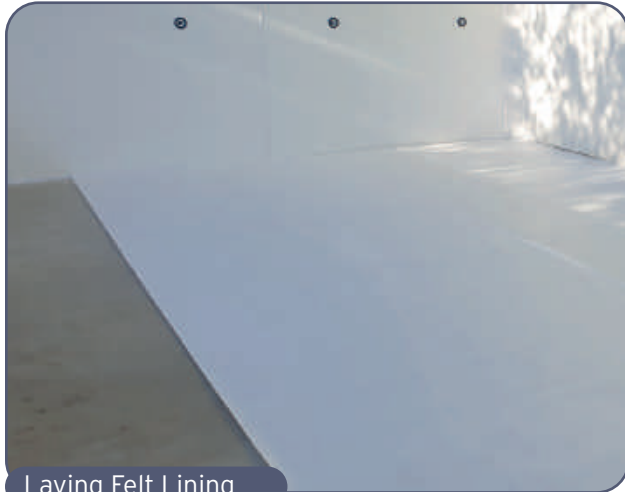
Laying Felt Lining
