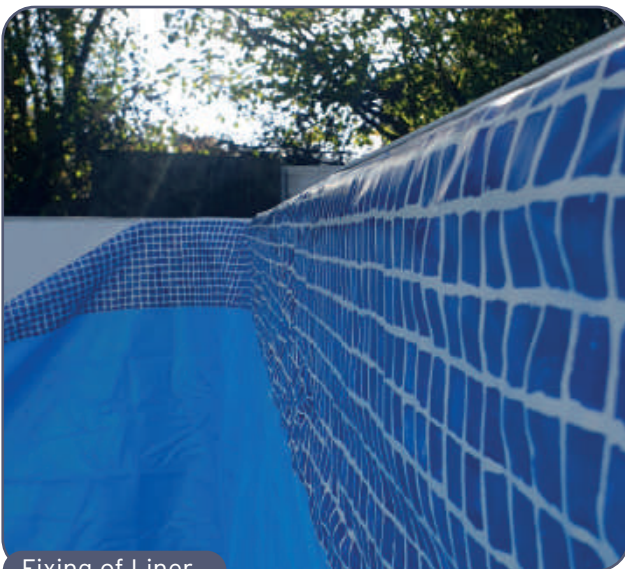
Fixing of Liner
